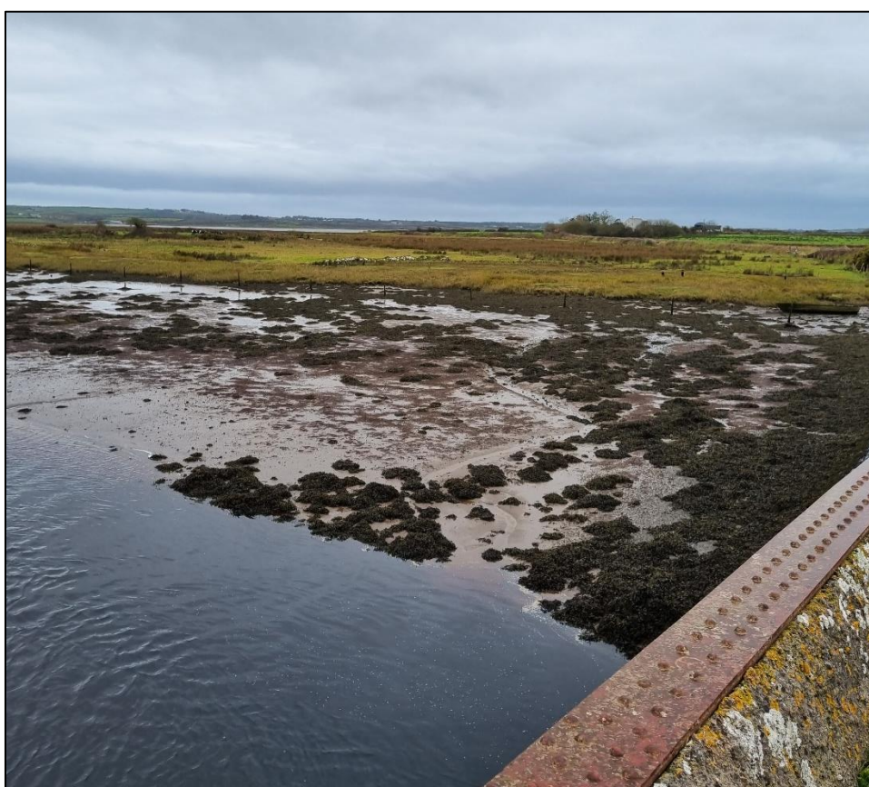
Plate 4.4 View off Moyasta Bridge looking west.
