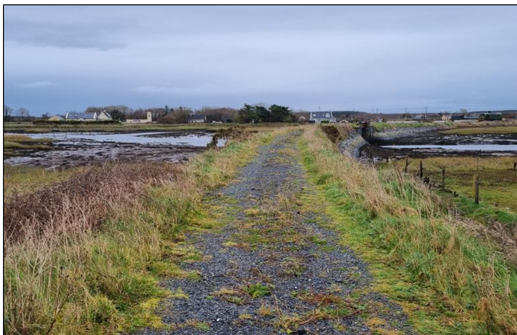
Plate 4.2 Ch. 7+750 looking east over Moyasta Bridge.
