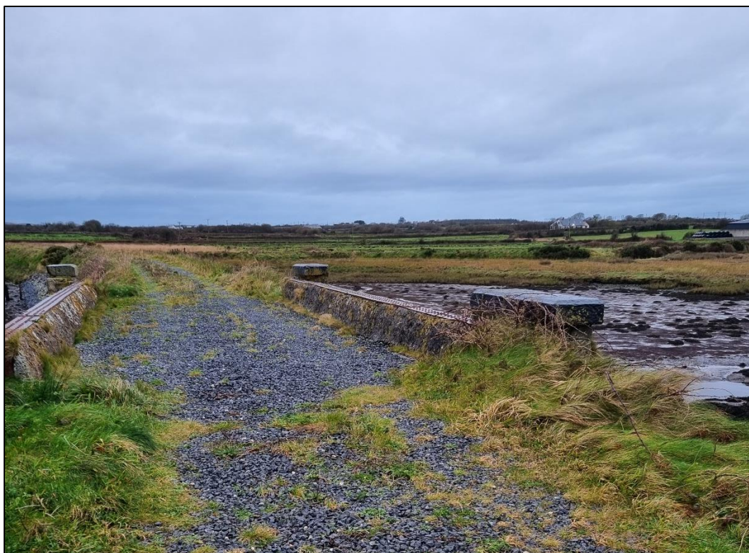
Plate 4.3. View west over Moyasta Bridge
